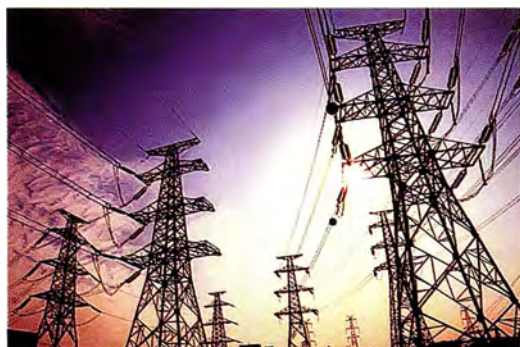
Electrical transmission towers are no match for a powerful solar storm.
